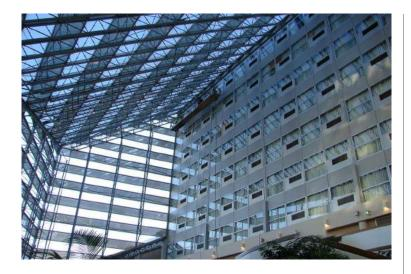
The main atrium of South Bend Marriott joins two separate buildings. These buildings rise several stories above grade. The space between the two buildings is covered by a large slope glazing system that is approximately 90 feet high at its highest elevation.
